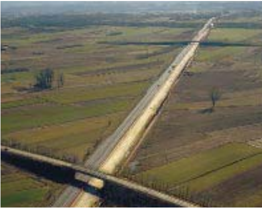
Torino-Savona motorway: doubling works on the Fossano-Mondovi section
