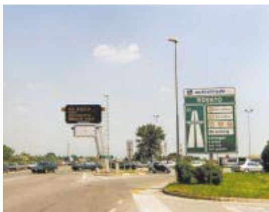
New digital message panels on the Milan-Brescia motorway
